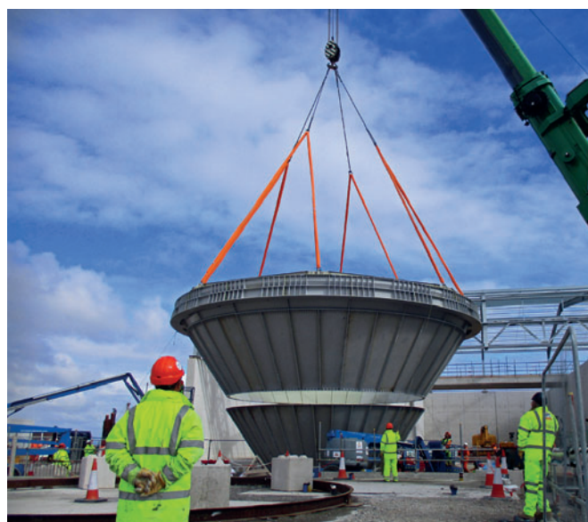
Construction of the base cone for the ground granulated blast furnace slag (GGBS) silo (April 2017). Image courtesy of EDF Energy 2017.
