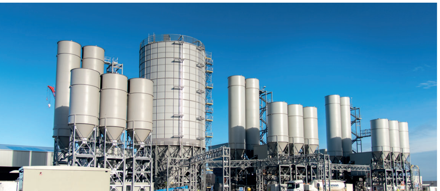
View of Bylor's three concrete batching plants, including a GGBS Silo at Hinkley Point C (December 2017). Image courtesy of EDF Energy 2017
