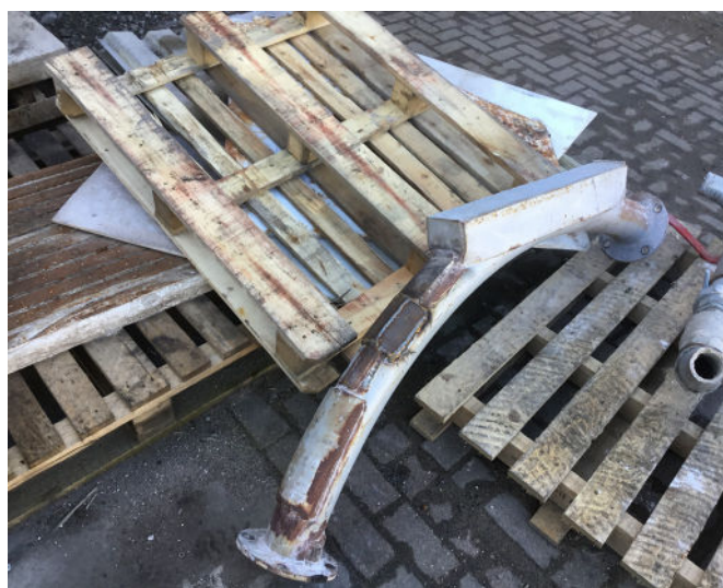
Remedial works on one of the steel pipes
