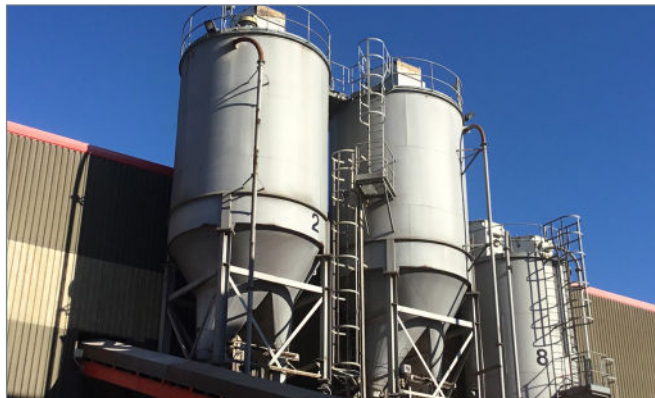
AlphaPipe installed to two plant silos
