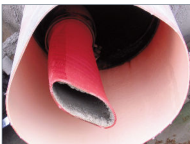
Conventional sleeves restrict flow
