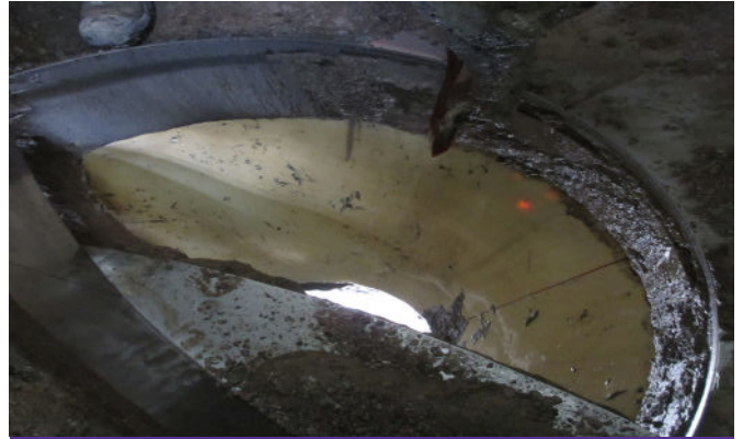
ConeFlex installation at CEMEX Widnes
