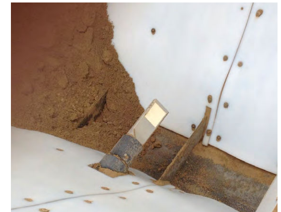
Hydronix probes installed in sand bins
