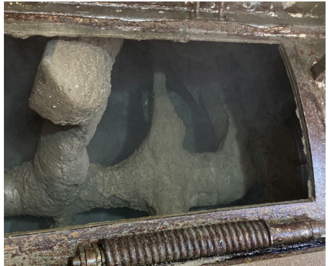
Concrete build-up in the single shaft mixer
