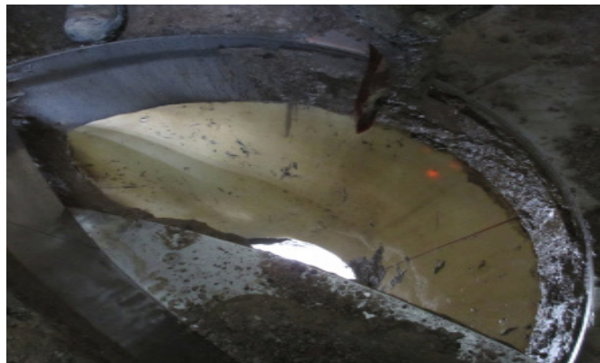
ConeFlex installation at CEMEX Widnes
