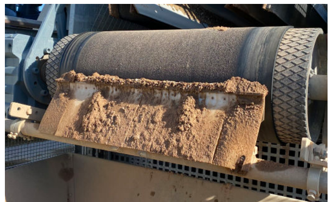
OEM scraper on the weigh belt overwhelmed with material
