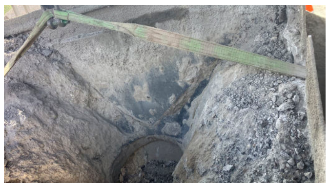
Discharge chute - removed, to chip out the build-up
